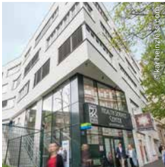
Health Service Center WIEN
